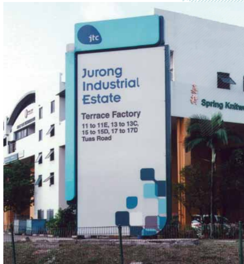
Jurong Industrial Estate, an area where there are many Japanese companies
